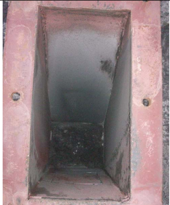
Photo 12 & 13: The effect of tack / stitch weld was seen very well in this chute, which was dismantled from position in boiler no2 during the visit. The weld beads had acted as nuclei for dust build up. Ideally the weld should not be present in the coal path.
